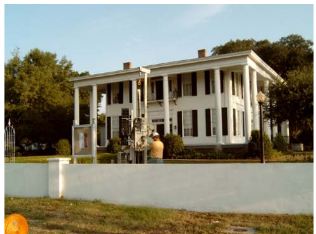
DTI injecting Cool-Ox™ Green
